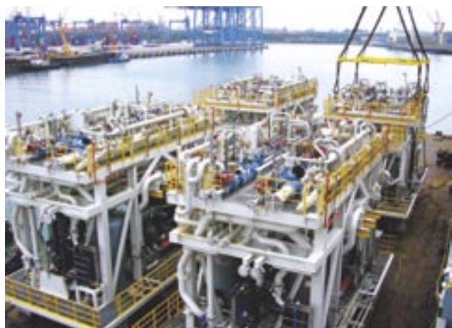
4 HP Modules on barge at Jurong Port, Singapore
