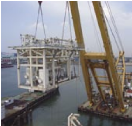
Stybarrow compressor being loaded
