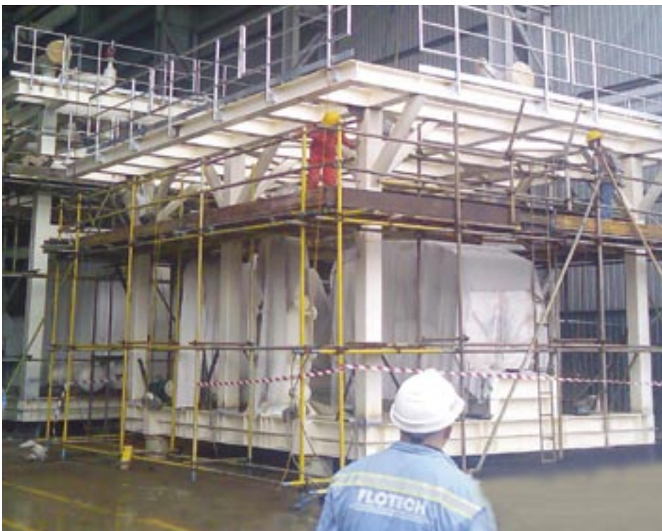
Stybarrow HP compressor frame at Singapore fabrication yard
